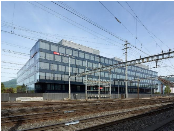
SBB Aarepark, Olten CFF Cargo et Infrastructure
